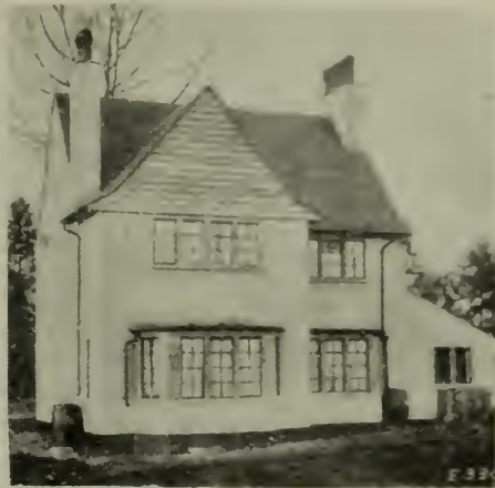
FIG. 8. A HOUSE AT CHALDON.
